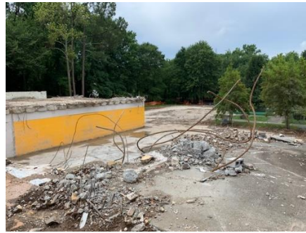
Demo of the vertical portion of the old school building complete
