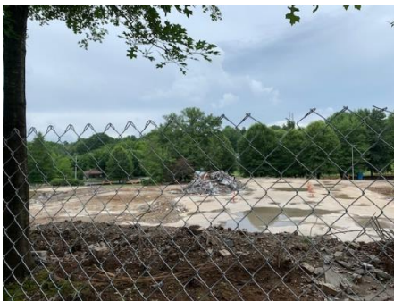
Demo continues on the existing School building
