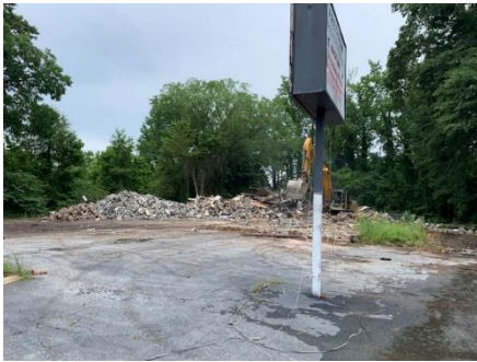
Transmission shop demo completed
